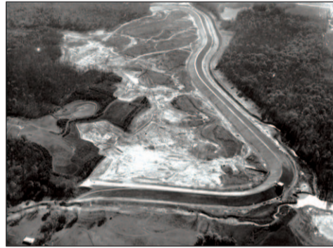
Construction of Lake Medina
